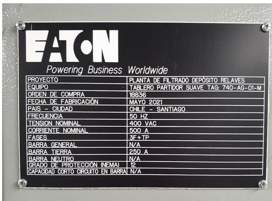
The image shows a black rectangular label with the Eaton logo and slogan at the top. Below the logo is a table with technical specifications for a soft starter. The table has two columns: the left column lists the parameter and the right column lists the value.
