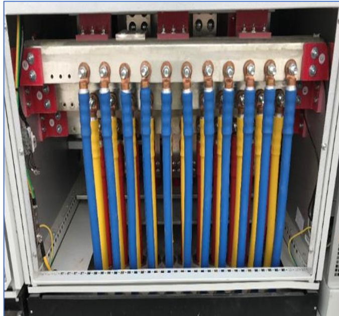
Figura 5.11: Cables AC.
